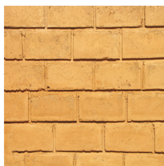
Compressed earth block infills
