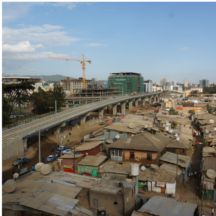
Light tram line
