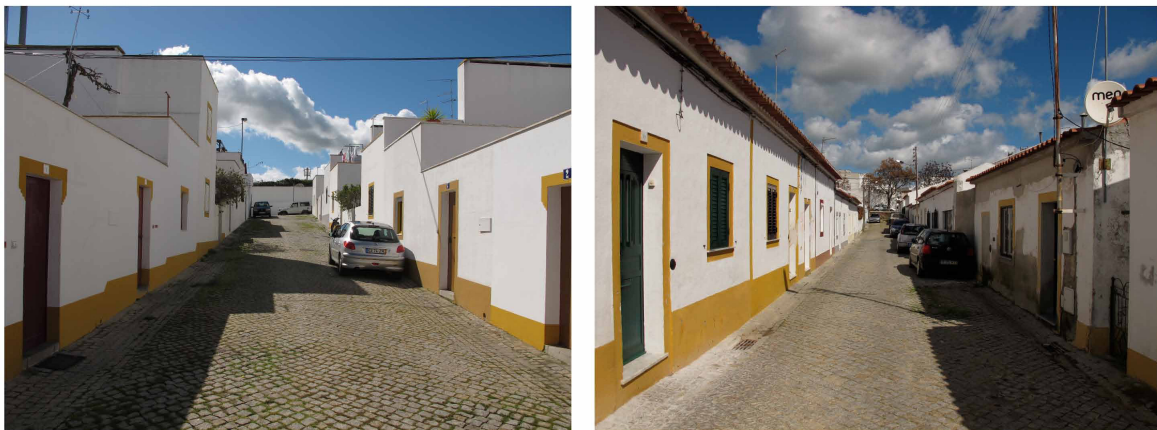
Figure 7: Current street views of the Malagueira neighbourhood (left), and the Clandestinos settlement - Bairro de S. Maria (right). Photos: © Nelson Mota.
