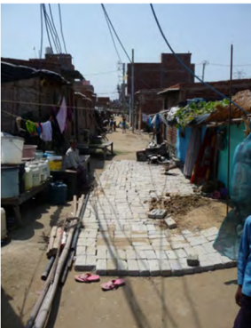
A typical half constructed road in block A
