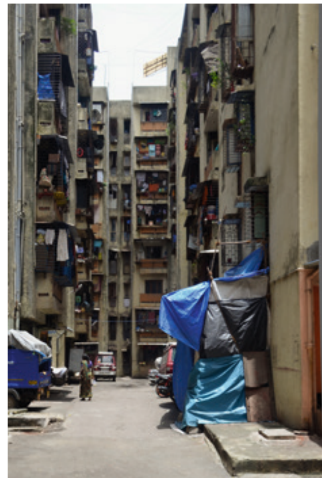
P.K. Das, Sangharsh Nagar Housing, Mumbai, foto: 2015 P.K. Das, Sangharsh Nagar Housing, Mumbai, photo: 2015
