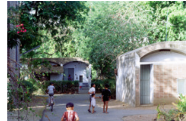
Balkrishna Doshi, ATIRA Housing, Ahmedabad, recente foto Balkrishna Doshi, ATIRA housing project, Ahmedabad, recent photo
