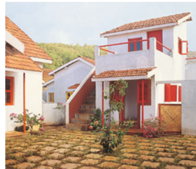
Charles Correa, Incremental Housing, Belapur, Navi Mumbai, 1986 Charles Correa, Incremental Housing at Belapur, Navi Mumbai, 1986
