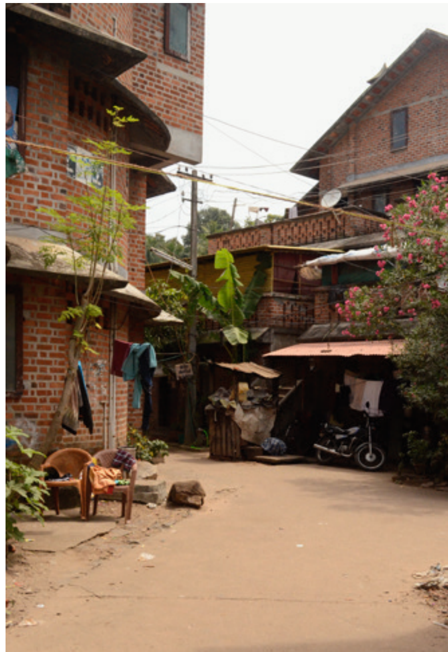
Laurie Baker, Chengalchoola Slum Development Housing, Trivandrum, foto: 2015 Laurie Baker, Chengalchoola Slum Development Housing, Trivandrum, photo: 2015
